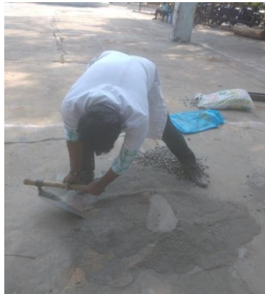
Figure 5 – Mixing of Concrete Manually
