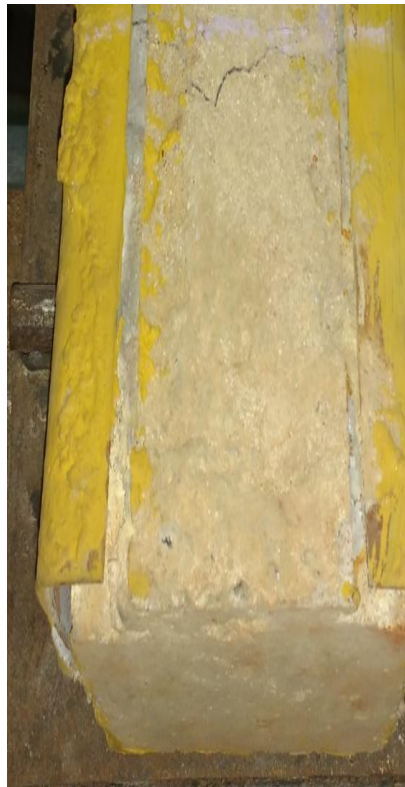
Figure 22- Crack and Separation of Steel from Concrete in CBT2
