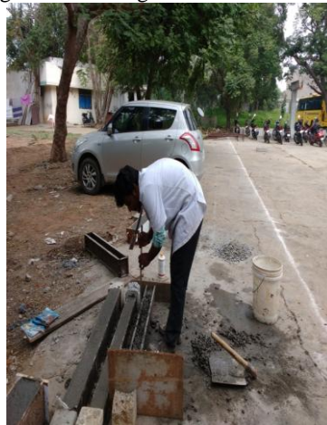
Figure 6 – Casting of Concrete
