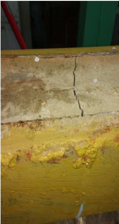
Figure 21- Flexural Crack of Beam CBT1
